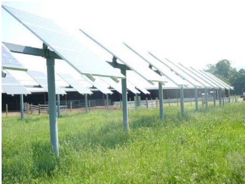
Testing height and spacing variations for growing pasture crops UMASS Amherst & NREL
